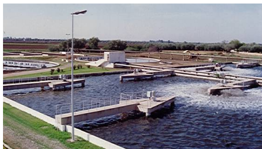
Figure 27 : Station d'épuration de Beni Mellal
